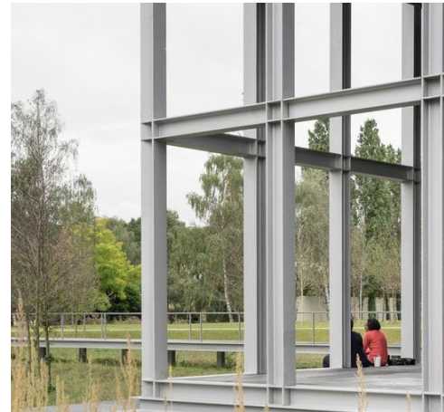
Steel facade structure
